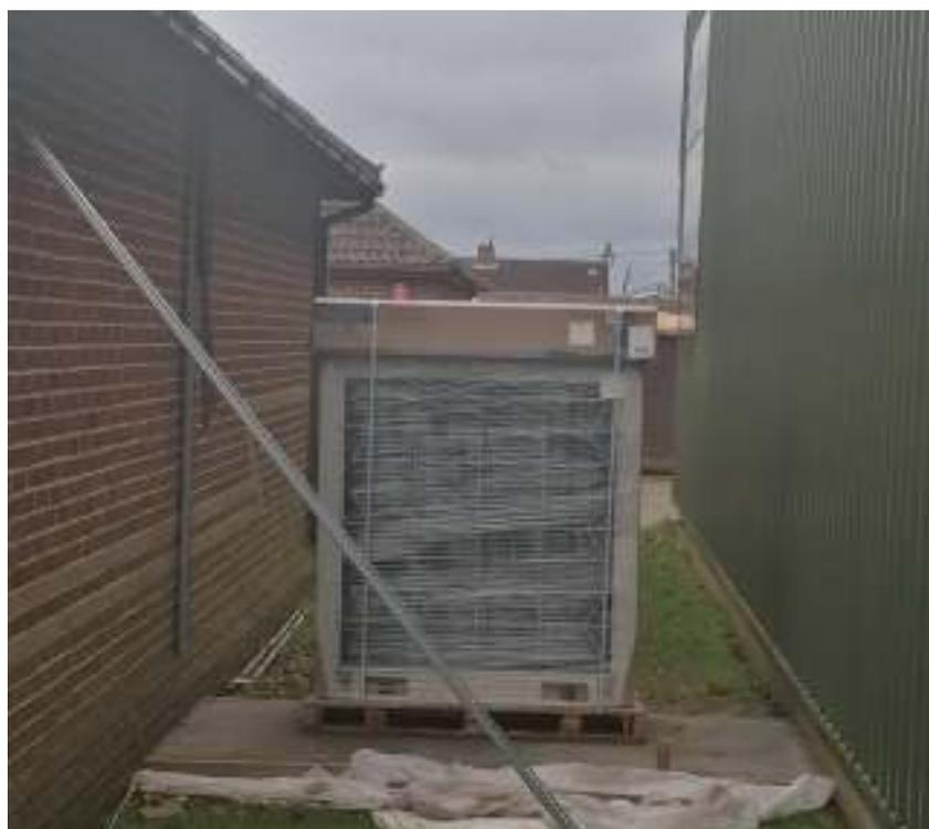
*The new main HVAC unit about to be installed, which will draw in the air from outside, this will then be heated, distributed around the building via a series of ducts and grilles.*
