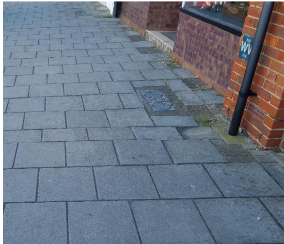
Further sunken/uneven paving outside NM Electrical & Simon@No11
