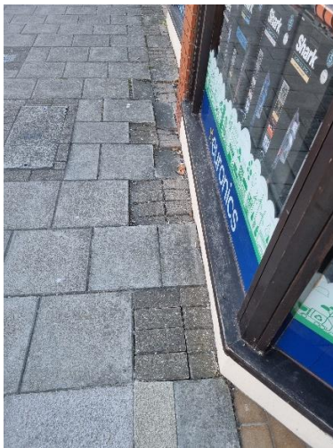
Further sunken/uneven paving outside NM Electrical & Simon@No11
