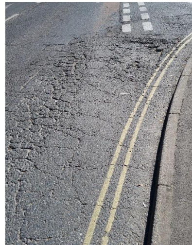
Long stretches of uneven paving between Simon@No11 & Buckgi Mini Market
