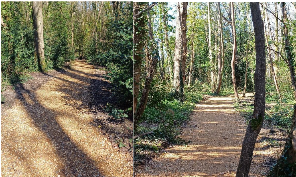
The completed gravel footpath at Carrick Wood
